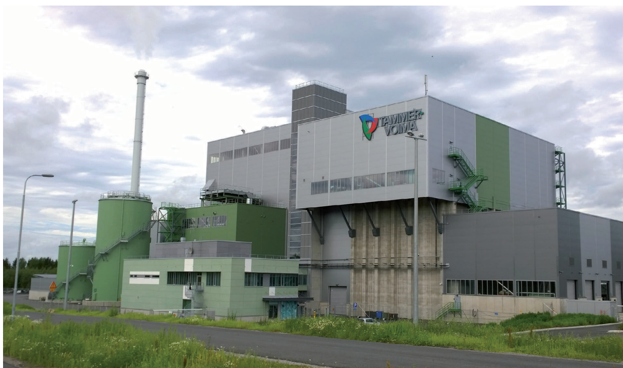
The Tammervoima waste-to-energy facility.
